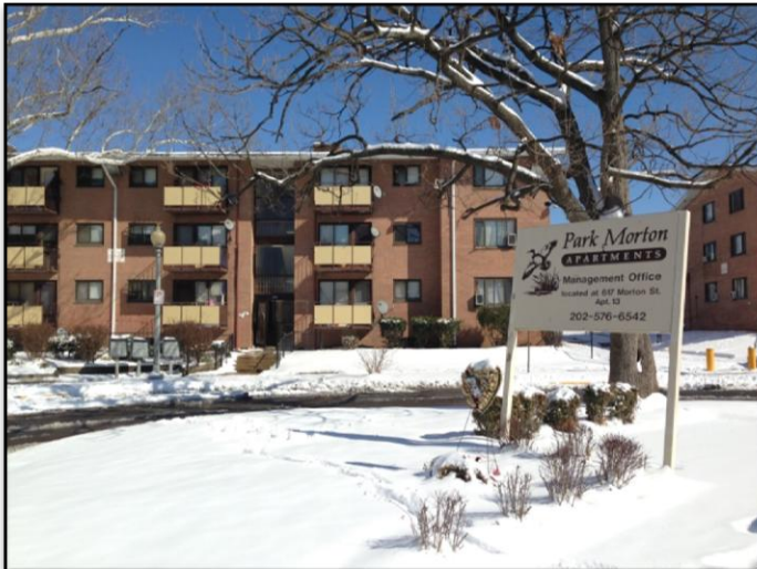
The Park Morton Housing development currently stands partially empty, fostering crime and blight rather than economic development
